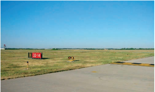
Holding position for Runway 14-32 on Taxiway Bravo. An above ground runway guard light is installed between the holding position sign and pavement marking.
